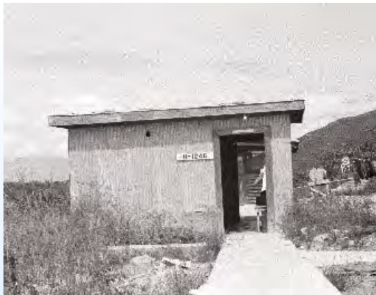
The Shower Building
