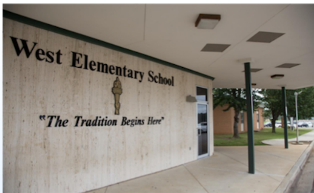
West Elementary School, Russellville, AL
